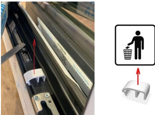
Fig. 7. Sash spacer shims:
